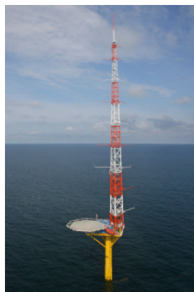
Figure 1: Offshore measurement platform FINO3
